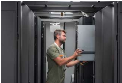
Private Network Construction & Maintenance
